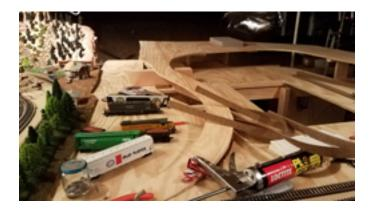
After attaching a sheet of 1 inch plywood, I started building the platform supports. I then cut a piece of 1/2 inch plywood for the track sub platform.
